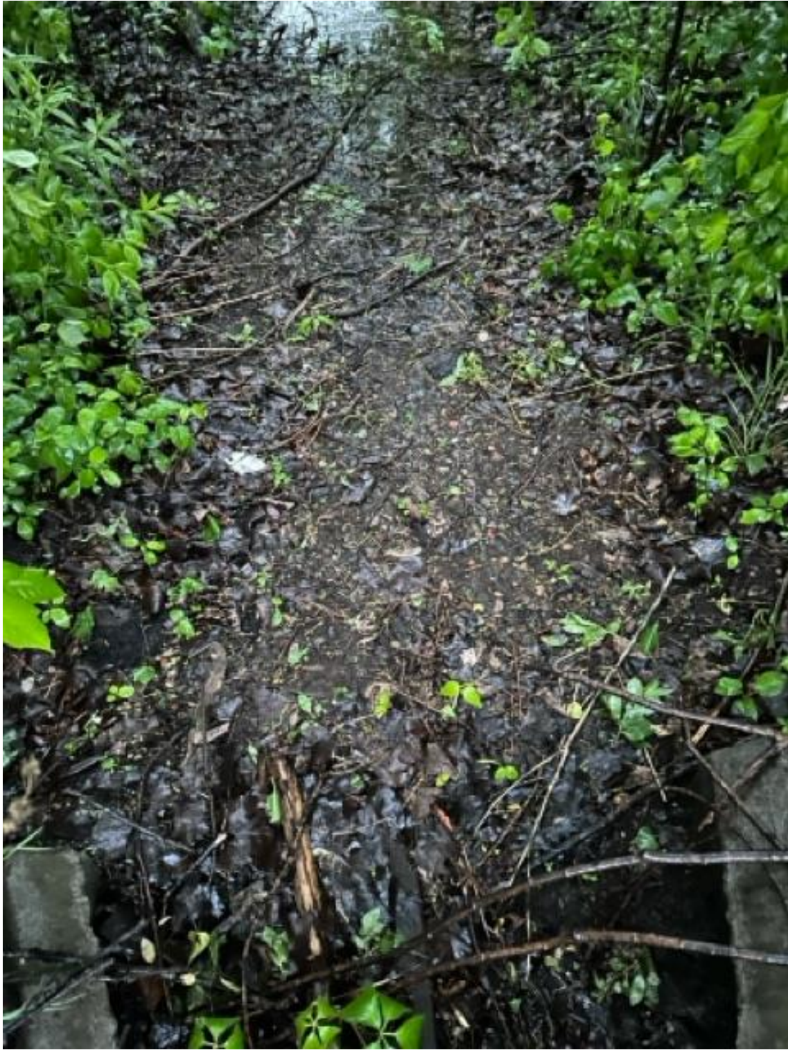
Picture taken from the culvert facing north. It is apparent that water is not flowing into the culvert.
