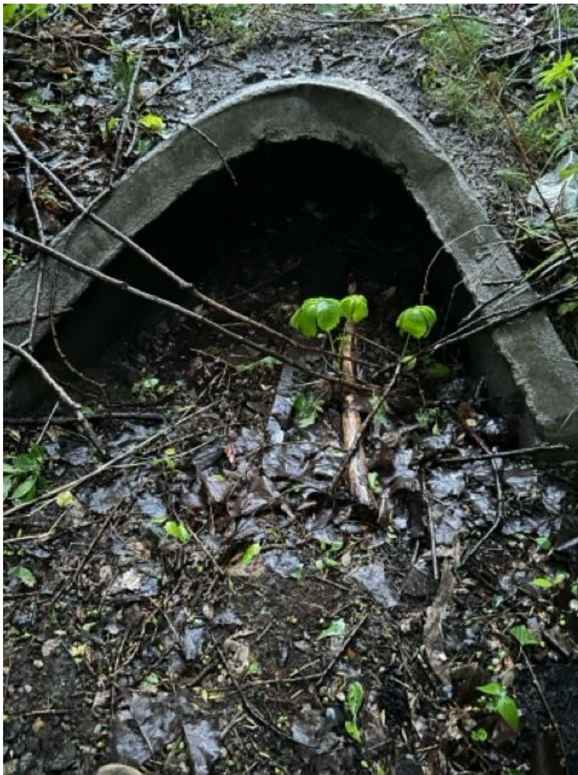
Picture taken of the culvert facing north. The culvert is unobstructed.
